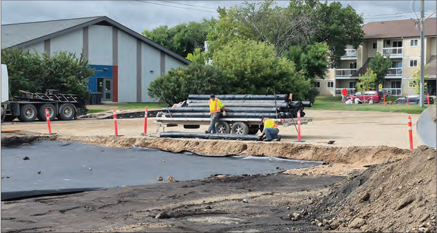
PHOTOS BY EOIN DEVEREUX The southwest section of the Yellowhead Centre's parking lot received upgrades recently, as new underground cloths were placed to assist in preventing frost boils each spring.
