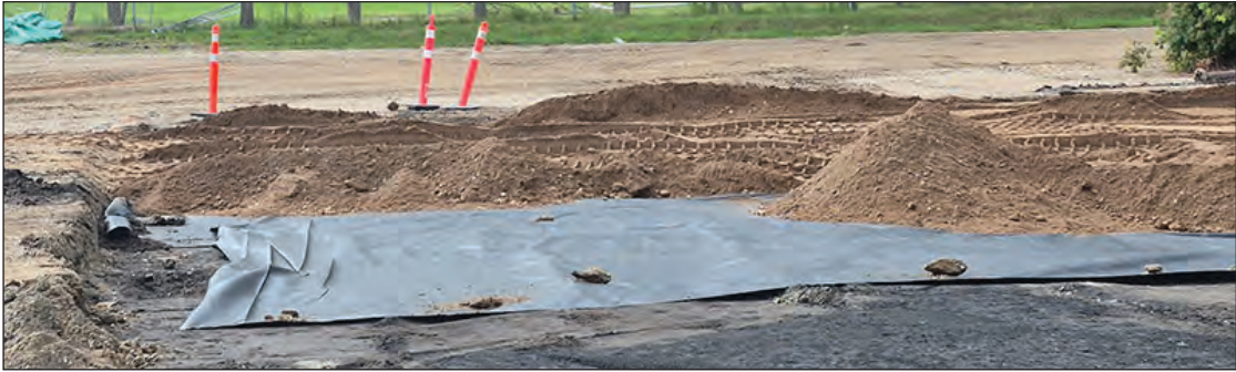
PHOTOS BY EOIN DEVEREUX The southwest section of the Yellowhead Centre's parking lot received upgrades recently, as new underground cloths were placed to assist in preventing frost boils each spring.
